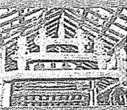
Stepped truss (梯步桁架)
