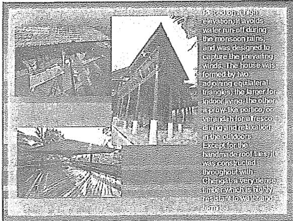
Placed on a high elevation it avoids water run-off during the monsoon rains, and was designed to capture the prevailing winds. The house was formed by two adjoining equilateral triangles, the larger for indoor living, the other a porch-like portico or veranda for al fresco dining and relaxation in the outdoors. Except for the handmade roof tiles, it was constructed throughout with Chengal, a very dense timber which is highly resistant to water and termites.
