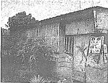
**Figure 58: Bamboo as Screen Material**
